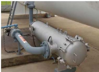
wave-shaped pleat geometry. This allows the use of significantly fewer elements and smaller housings, which is particularly beneficial in bulk diesel fuel applications where high flow rates and high contamination ingress rates are present. Ultipleat diesel fuel housings have been designed so that all sizes use the same installation footprint. This allows users to easily replace a smaller housing with a larger one - with no costly pipework modifications - should process changes
